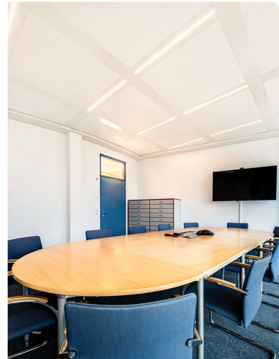
Air-conditioned ceiling with integrated lighting
