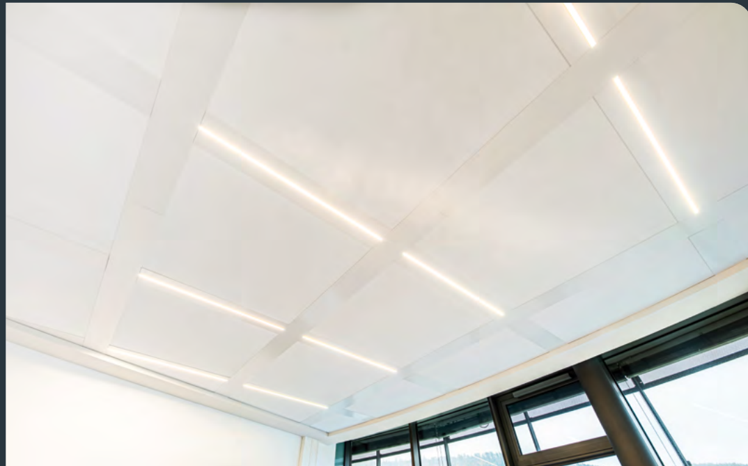
Climate ceiling with integrated illumination
